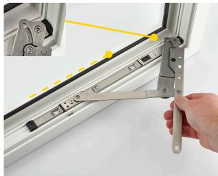
1. Position the hinge onto the frame and push the head of the hinge into the corner as shown.
