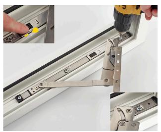
5. Slide the "Easy Clean" activation button and move the top slider until final screw position is exposed and insert countersunk screw\*. **Important note:** Variant 0115-2008 does not have an easy clean funcion.
