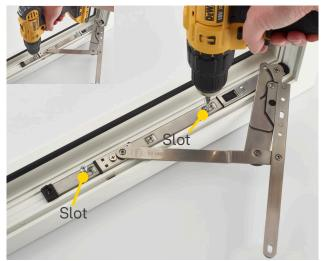
2. Insert 2 countersunk screws\* into the slots shown. The screws must be positioned at end of the slot, furthest from the head of the hinge as shown.
