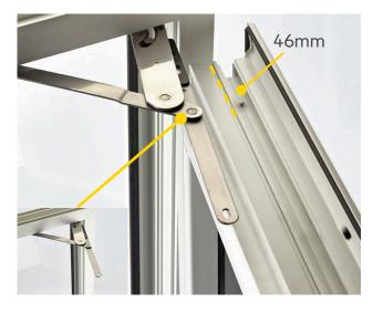
46mm is the distance from the edge of the Sash rebate to the middle of the first slot on the Sash.
