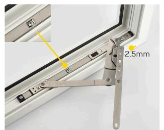
3. Slide hinge out so that screw is seen in the centre of slot leaving 2.5mm for adjustment if required.
