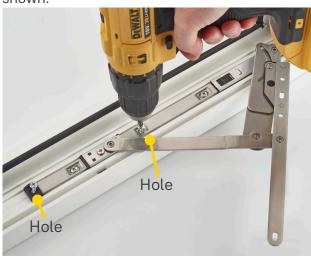
4. Insert countersunk screws\* into the 2 screw holes as shown.
